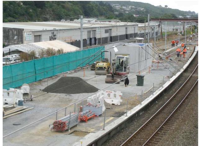
New drainage has now been installed on the platform and this should prevent pooling.
